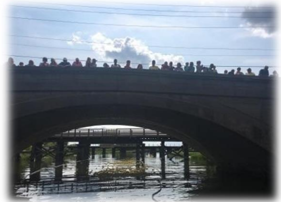
"View of bridge from one of the pontoons"
